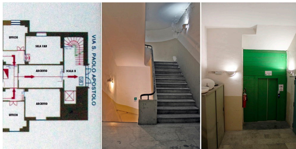
Figure 12. The transformations of the 1970s: one of two mixtilinear stairs is demolished to make way for an elevator.
