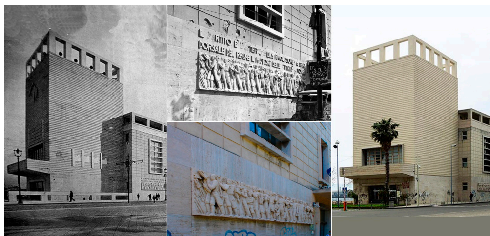
Figure 13. The transformations of the 1980s: the plastering of the travertine tower.
