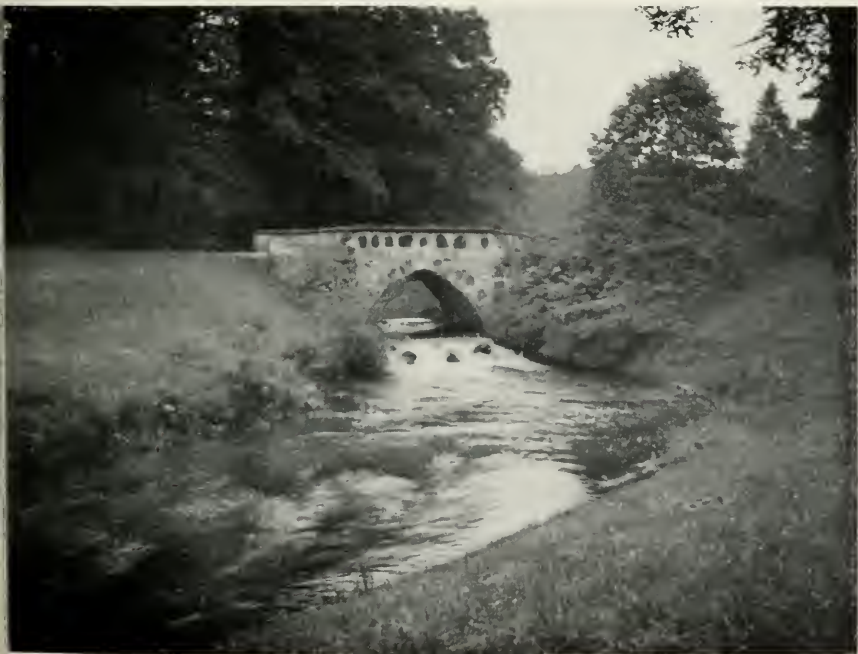
A Rough Stone Bridge in the Park on the Estate of Prince Pückler von Muskau. From a Photograph by Thomas W. Sears, Providence, R. I.
