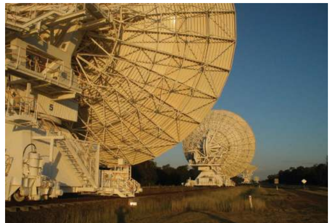
Figure 2. The ATCA. Displayed are several antennas on the east–west track pointing at a source near the horizon.
