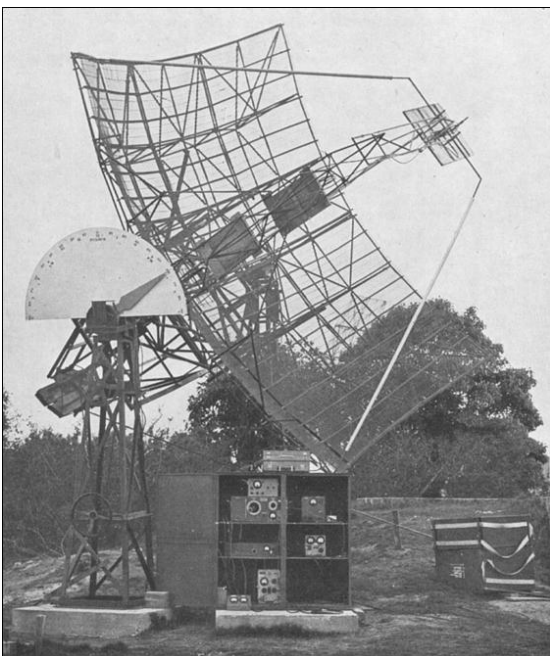
Figure 2: The 16 x 18-ft paraboloid at Georges Heights field station. It was proposed to ship this aerial to Brazil for the 1947 total solar eclipse (courtesy ATNF Historical Photographic Archive: B1164).
