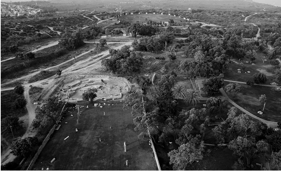
FIG. 6. Aerial view of the excavation area, view to the southeast toward the theater and ramparts.
