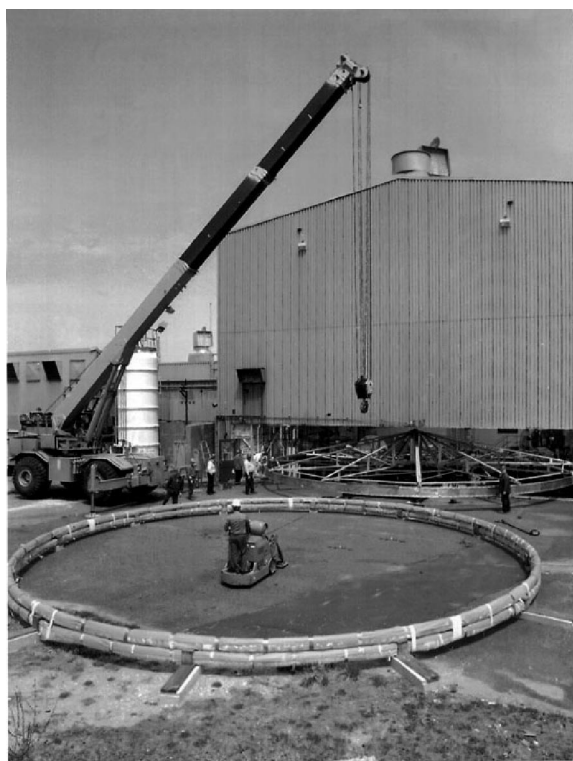
Fig. 6. The completed outer coil and cryostat were passed through the slot in the g-2 building and stored outside, in preparation for construction of the lower half of the magnet yoke. The completed inner coils in their cryostats are in the foreground.
