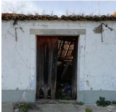
Figure 4: Caramela dwelling detail of iron stabilising rods in Vale da Vila, Pinhal Novo, Palmela, Portugal (2017)
