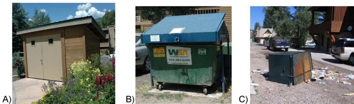
Figure 2. Examples of refuse collector designs. Designs that are considered bear-proof in the city of Aspen and the surrounding residential area of Pitkin County including: A) A low-risk dumpster room with metal doors, round handle, and little door clearance, B) a medium-risk dumpster with bolted, metal lid over a free-standing dumpster, and C) a high-risk free-standing dumpster with top-bar securing method that was toppled and broken into by a bear.
