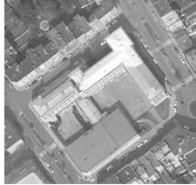
Figure 3: Aerial image of high resolution with a school building and surrounding streets.
