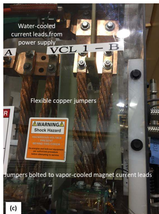
Figure 47: (a) Screen shot of vacuum pumping control screen for the torus, (b) Distribution can being delivered to Hall B, (c) Flexible copper jumpers connecting the torus water-cooled leads to the magnet vapor-cooled leads.
