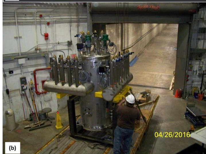
Figure 47: (a) Screen shot of vacuum pumping control screen for the torus, (b) Distribution can being delivered to Hall B, (c) Flexible copper jumpers connecting the torus water-cooled leads to the magnet vapor-cooled leads.
