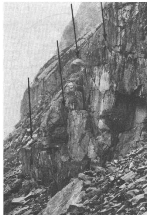
Fig.6. Toppling failure in Nant Peris; destabilization caused the parting of blocks along arrowed discontinuities.
