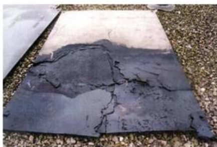
Figure 1. Catastrophic failure along barrier board [7]
