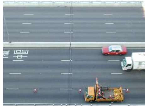
Fig. 15. Lane closure. Contractors are placing traffic cones to close the lane
