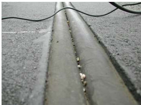
Fig. 4. The bridge movement joint on Bridge A
