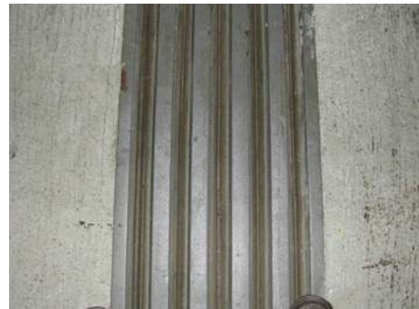
Fig. 6. The bridge movement joint on Bridge B
