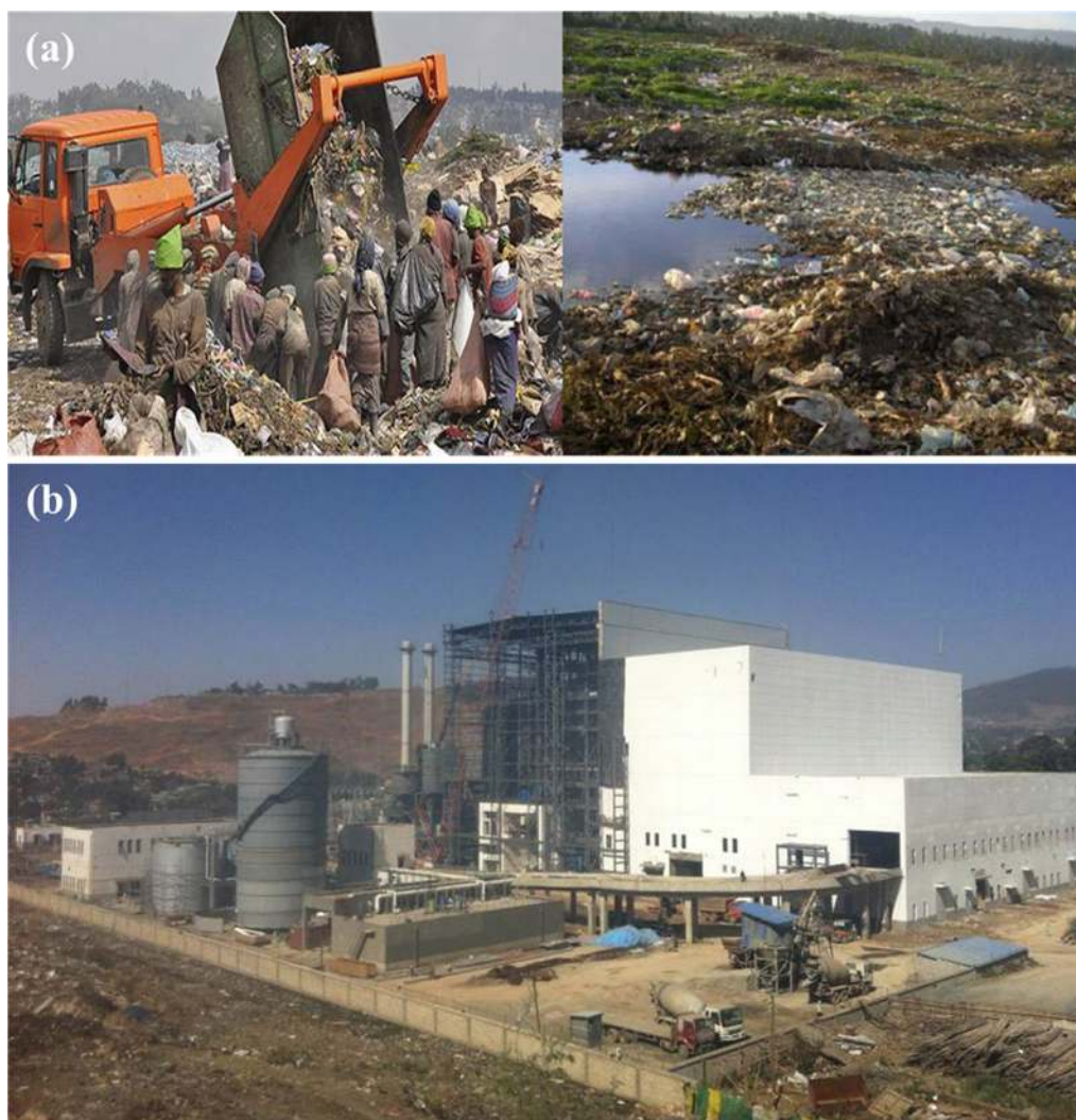
Fig. 10 a 'Reppi', solid waste disposal site and compaction; b 'Reppi' waste-to-energy power plant
