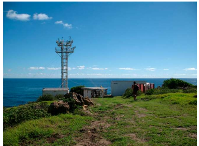
Fig. 11. The University of Miami Barbados Atmospheric Chemistry Observatory, Ragged Point, from 1989 to present. The aluminum walk-up scaffold tower is 17 m tall; the elevation of Ragged Point is 30 m. The structure at center and the one on the right are the University of Miami laboratories, converted 6-m ship containers. The building on the left is the laboratory of the Advanced Global Atmospheric Gases Experiment (AGAGE) program (Archibald et al. 2015; see the section “The impact of African aerosol transport on air quality” in the supplement). The view in the photo is to the northeast. See Fig. ES11 for other images related to site facilities.
