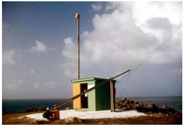
Fig. 10. The first University of Miami research facility located on the easternmost end of Ragged Point, 1971 (13.165040°N, 59.432070°W). The filter heads were located at the top of the fold-over masts. Several years later, the masts in the photo were replaced by a 10-m fold-over tower that was used until 1989.
