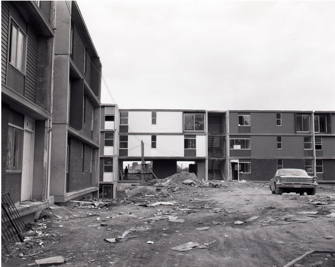
Figure 3.4: Construction of Academy Homes, 1967. (Image: Boston City Archives)
