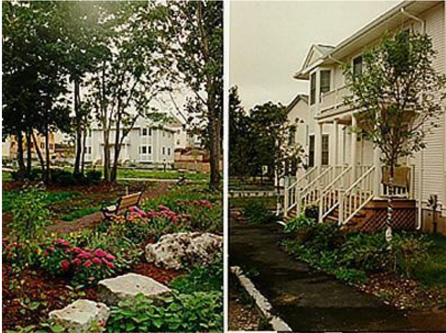
Figure 4.15: Winthrop Estates project area after construction. (Image: Dudley Neighbors Inc.)
