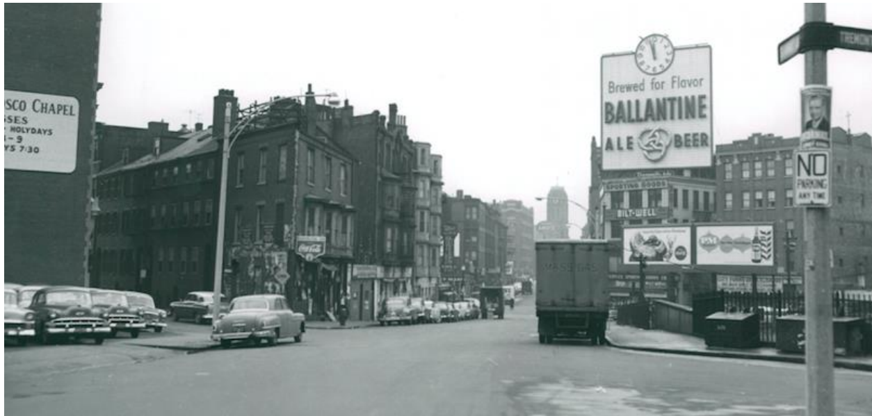
Figure 2.3: Intersection of Tremont and Shawmut Streets, 1952. (Image: Boston City Archives)
