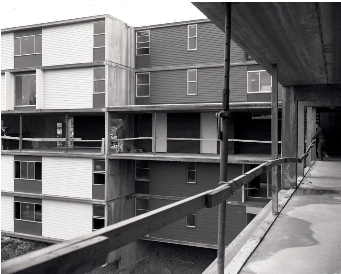
Figure 3.3: Construction of Academy Homes, 1967. (Image: Boston City Archives)
