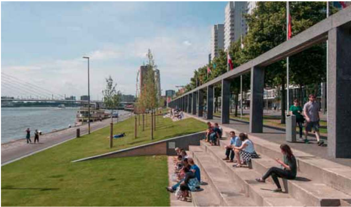
Fig. 2 View of Boomjeskade in Rotterdam. The impermeable pavement of the riverbank was replaced with grass creating a soft infrastructure for flood buffering that at the same time serves as a green space for people to use. (Photo: Gemeente Rotterdam 2013; authors' adaptations and editing)
