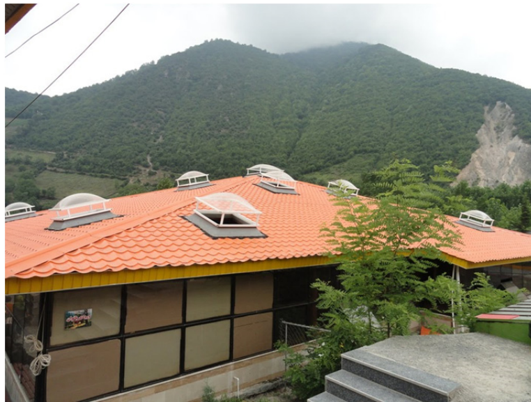
Figure 3. Lavij hot spring building
