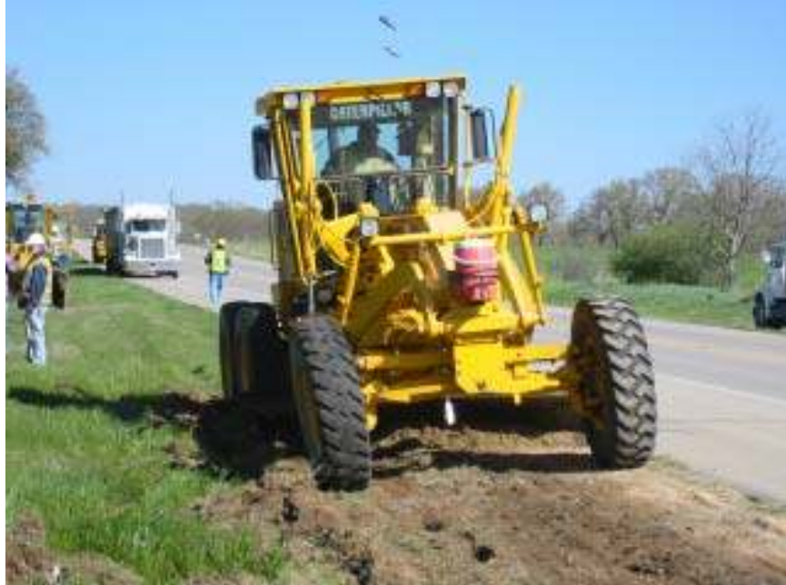
Figure 5.2 Maintainer to Blade the Subgrade Shoulder
