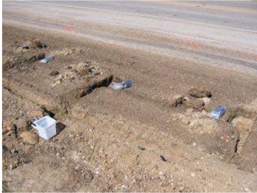
Figure 5.7 Placement of Sensors in a Test Section
