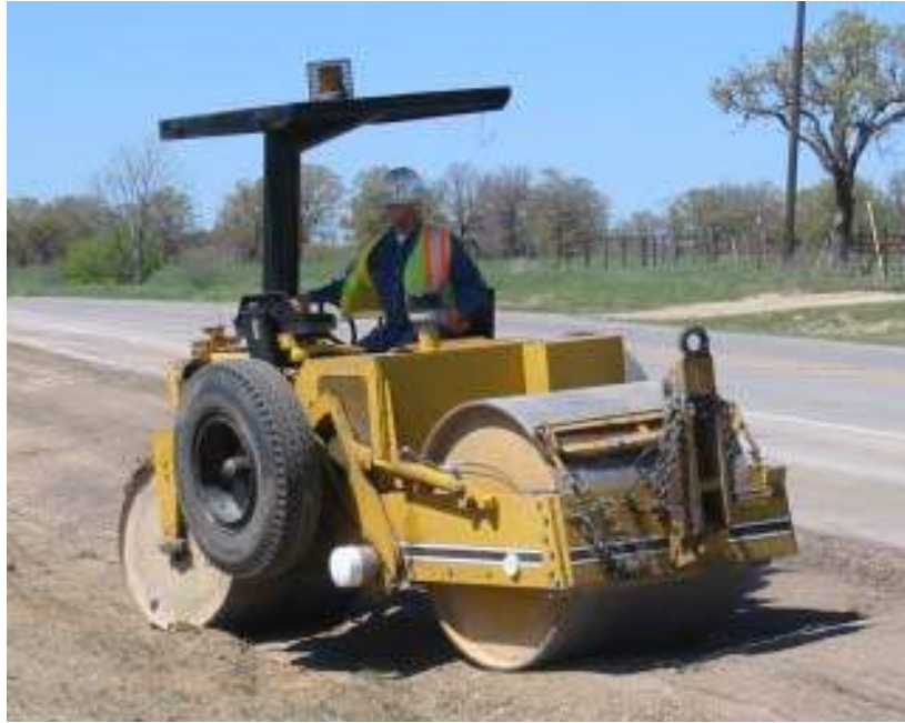
Figure 5.6 Smooth Drum Roller Used for Soil Compaction
