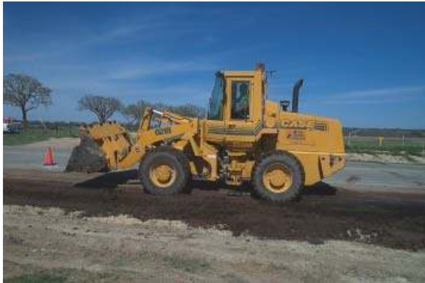
Figure 5.4 Distributing Composts on the Tilled Subgrade
