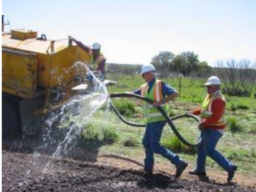
Figure 5.5 Application of Water over the CMT Loose Mixture
