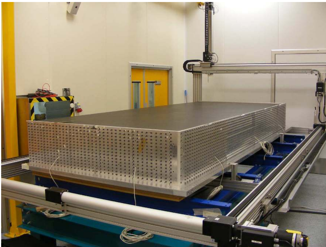
Figure 3. One of the top barrel-ECal 1.5 \text{ m} \times 4 \text{ m} modules lying horizontally during construction. The fibre ends encased in their ferrules are visible protruding from the module bulkheads. The structure of the 2D scanner can be seen surrounding the module.
