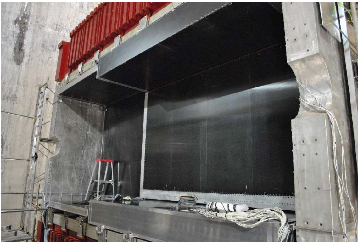
Figure 2. One entire side of the ECal in situ installed in the ND280. The three P0D-ECal modules are on the left in the figure, the three barrel-ECal modules are on the right. Part of the magnet yoke (top, red) is visible.
