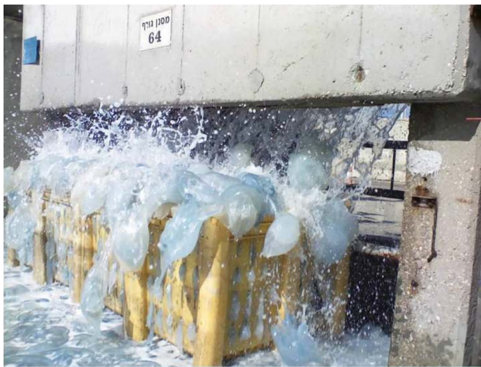
Fig. 3. A swarm of the scyphozoan jellyfish, Rhopilema nomadica , likely introduced through the Suez Canal, blocked water-intake pipes of power plant in Israel, 2011.
