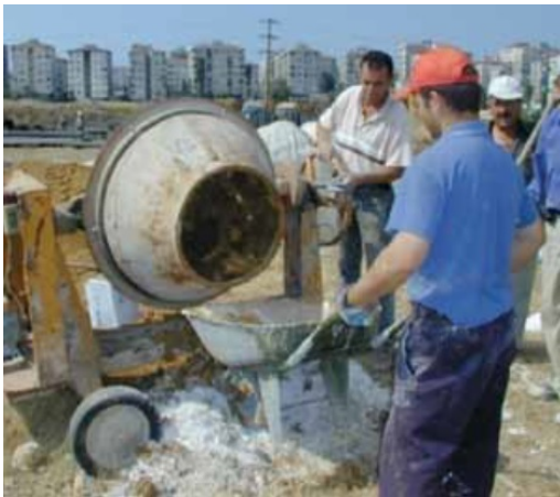
Fig. 2. Preparation of adobe block with gypsum [38].
