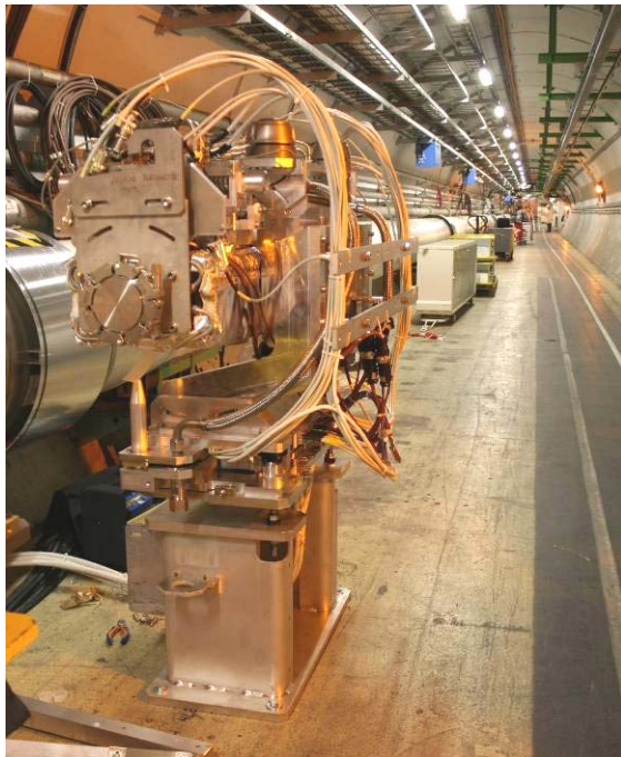
Figure 6: Photograph of an installed ring collimator on its quick plug-in support in IR8 of the LHC.
