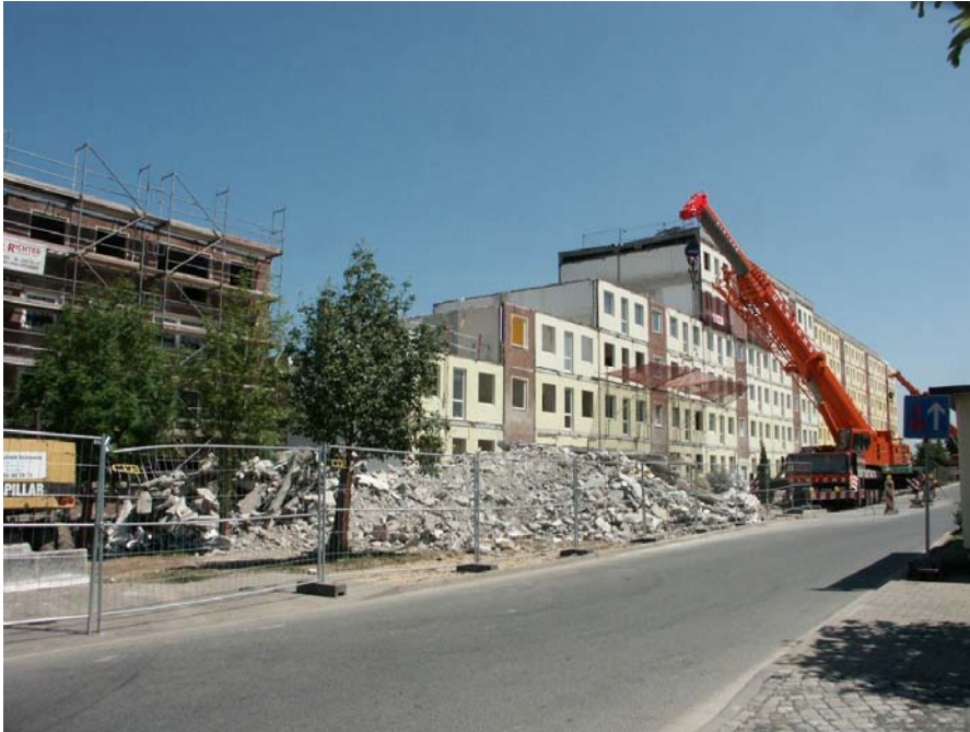
Figure 4: Deconstruction of large housing blocks in Dresden (Photo: IOER)
