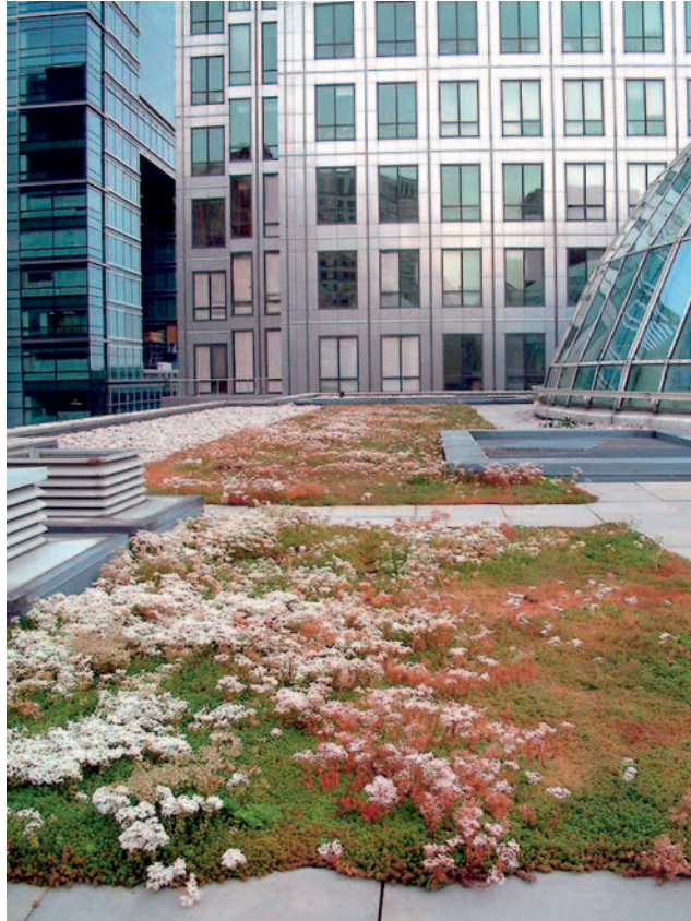
Fig 1 | Retail sedum roof, Canary Wharf, London, UK. Reproduced with permission from Kadas, 2006.
