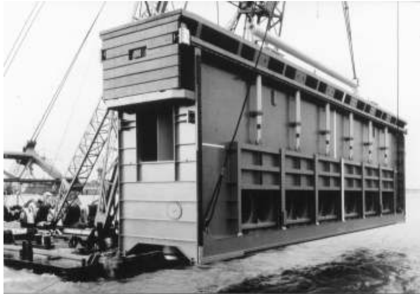
Figure 2.2: Placing of a lock-gate in the PWA-lock.
