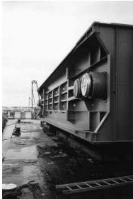
Figure 2.3: Bottom of the lock-gate. The hydro-foot and the fixed foot closest to the camera are clearly visible.
