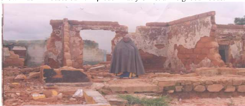
Plate 1: A House Burnt in Jos South, (Field Survey, 2011)
