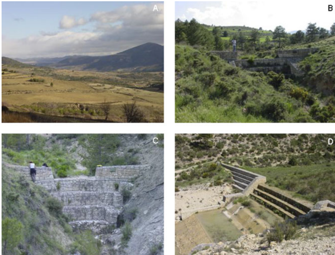
Figure 2. (A) General view of the catchment in November 2004; (B) check-dam in a tributary river at the medium catchment in May 2004; (C) check-dam in a tributary river at the upper catchment in June 2004; (D) check-dam at the outlet of the catchment in May 2005
