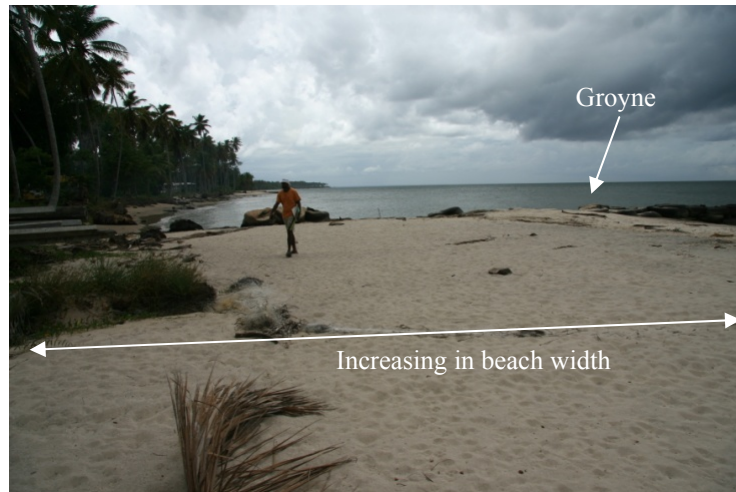
Figure 18. Visible sediment impounding updrift of groyne 2 at station 3, modifying the shape of the coastline (25th September, 2009)
