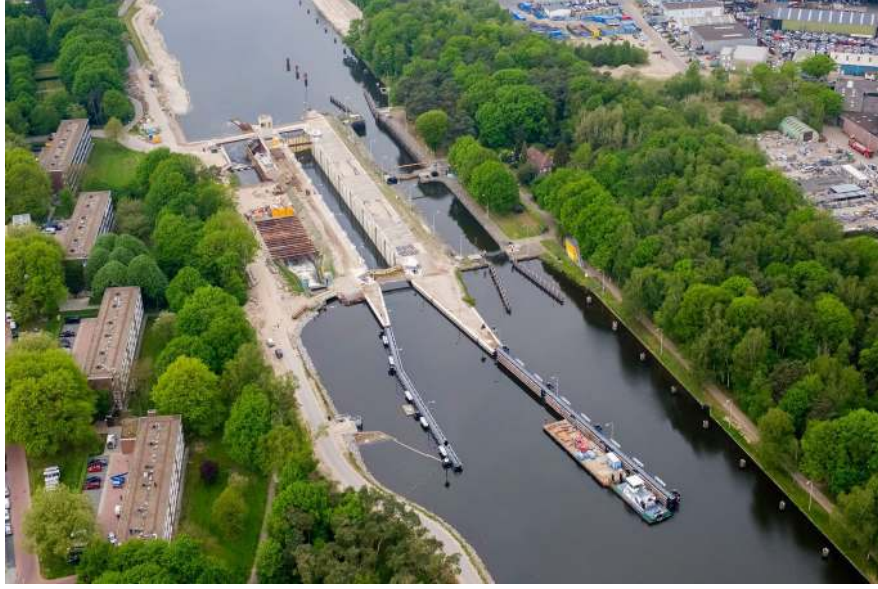
Fig. 3. Photo of Lock III, located at Tilburg, The Netherlands. Image from https://beeldbank.rws.nl , Rijkswaterstaat.
