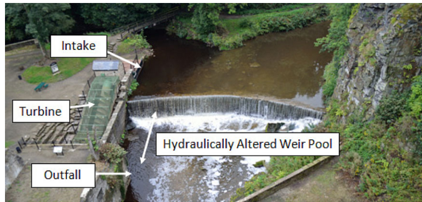
Fig. 2. An example of a low-head in-weir scheme (Torr's Hydro Scheme, New Mills, Derbyshire, UK).
