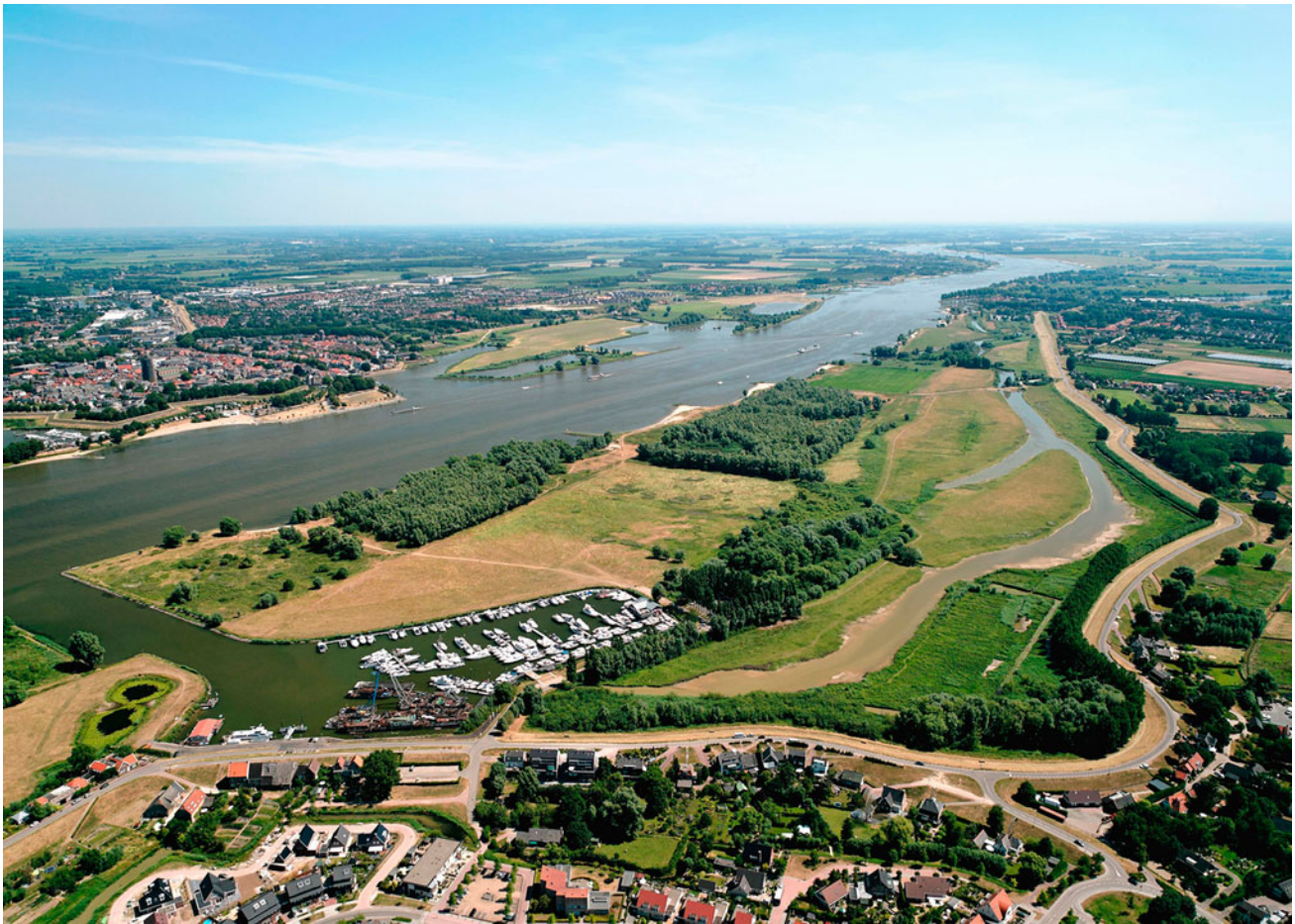
Fig. 1 Aerial view of an embanked floodplain with a mosaic of woodlands and grasslands along a Rhine distributary in the Netherlands. View looking upstream. The winding road on the foreground
