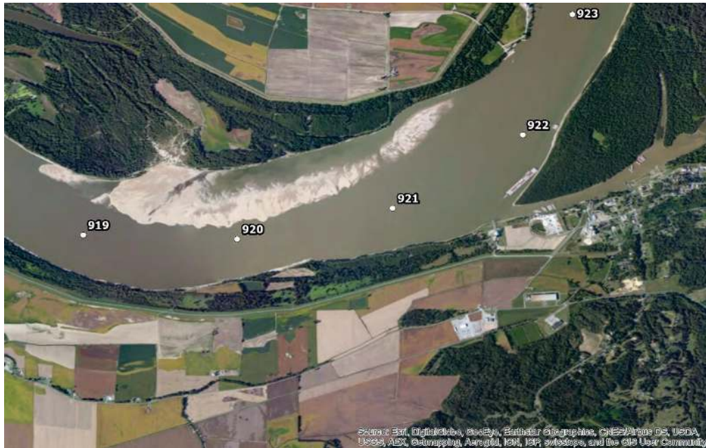
Figure 15. Aerial view of the Hickman area. Scour pool is between RM 920 and RM 921.
