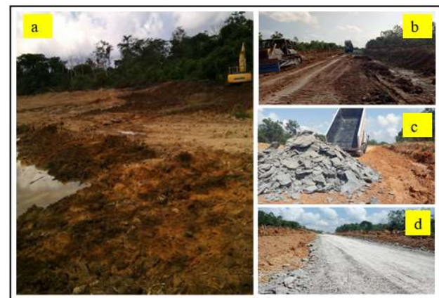
Figure 11: Preparation of connecting road from pit to phase 4 “layering road”.
