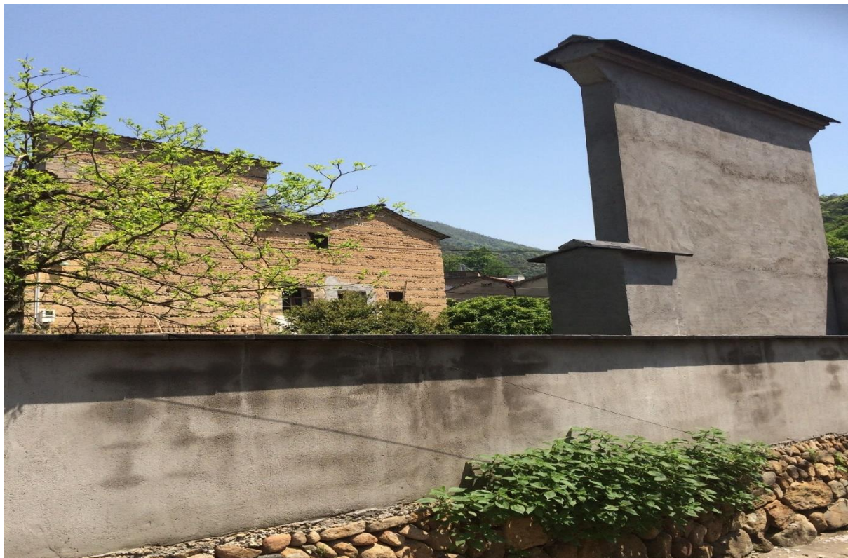
Figure 3: Cement wall in front of late Qing Dynasty house
