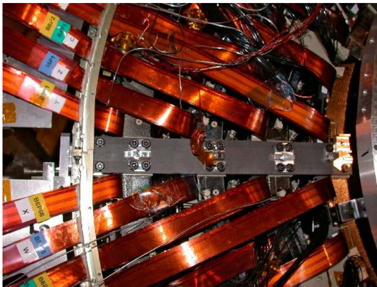
Figure 28. Photograph showing one of the 8 interlinks at one end, after the four barrel assembly.
