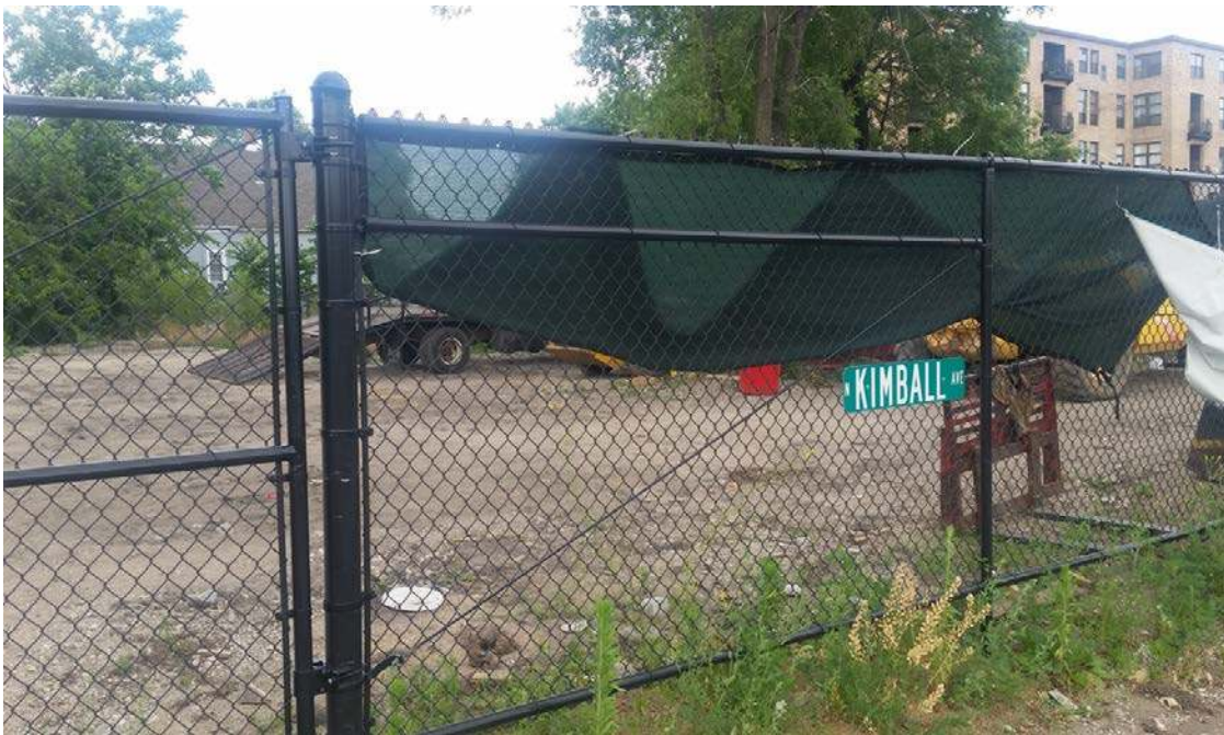
Figure 2: Image of an unfinished lot located directly off the paved surface of The 606 at Kimball Avenue.
