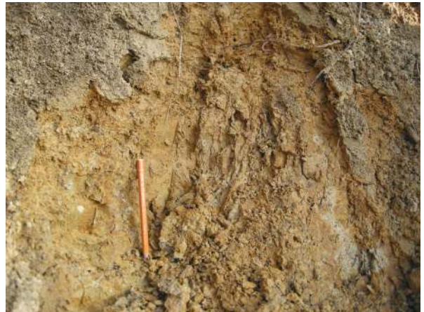
Fig. 9 - Pervasive N-S oriented fractures in the S. Martino Unit silt SE of Valfenera Village, referred to the T. Traversola Deformation Zone.
