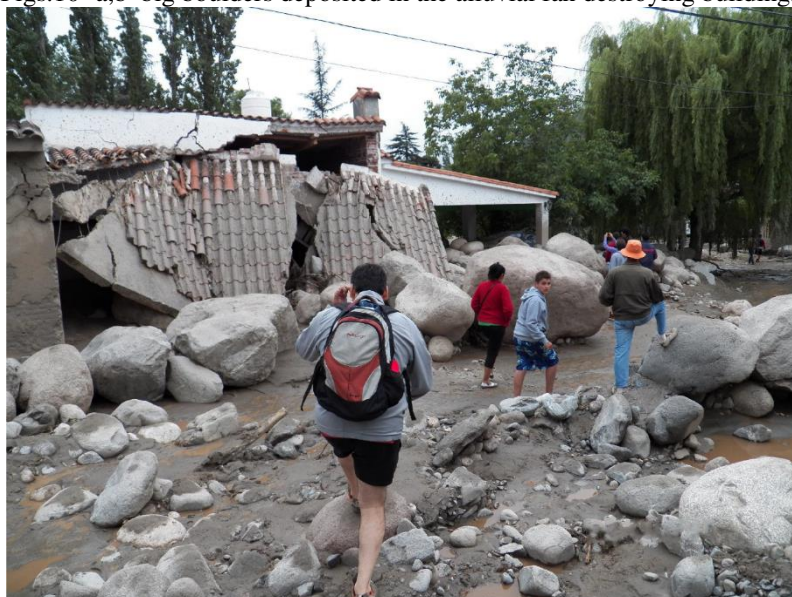
Figs.10- a,b big boulders deposited in the alluvial fan destroying buildings.
