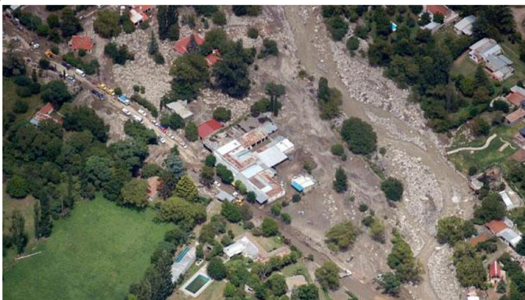
Fig. 14. Aerial view of the alluvial fan showing built areas in the floodplain damaged by the flood (El Esquiu newspaper, 25 January 2014)
