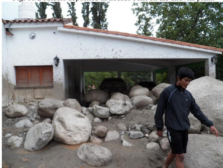
Fig. 11 Boulders deposited in houses built on the alluvial plain.
