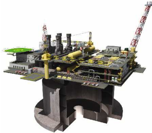
Figure 1. A mono-column, floating oil production platform. The risers and umbilical cables that connect the production plant to the well heads are suspended from the platform through the moon-pool.
