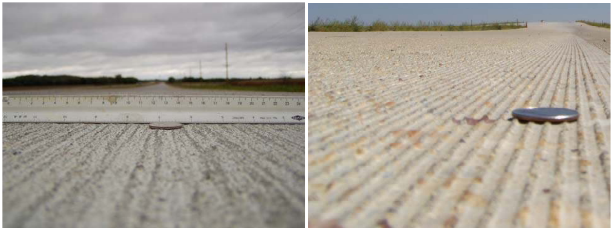
Figure 28. Drag and diamond ground concrete pavements (source: CP Tech Center).
