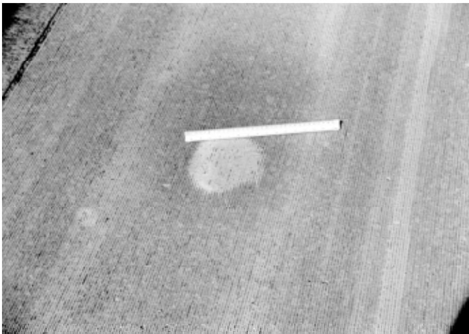
Figure 33. Sand-patch measurement for newly ground pavement.
