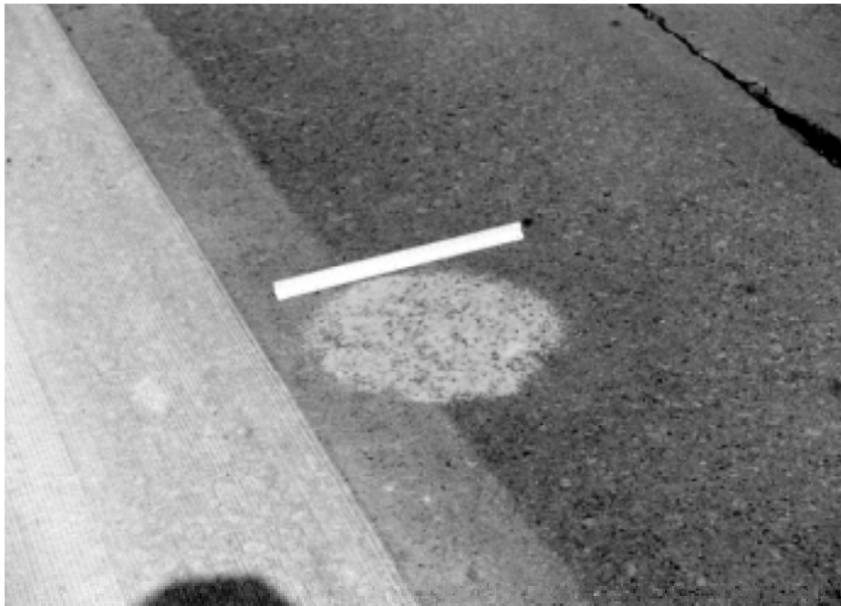
Figure 32. Sand-patch measurement for nonground pavement.
