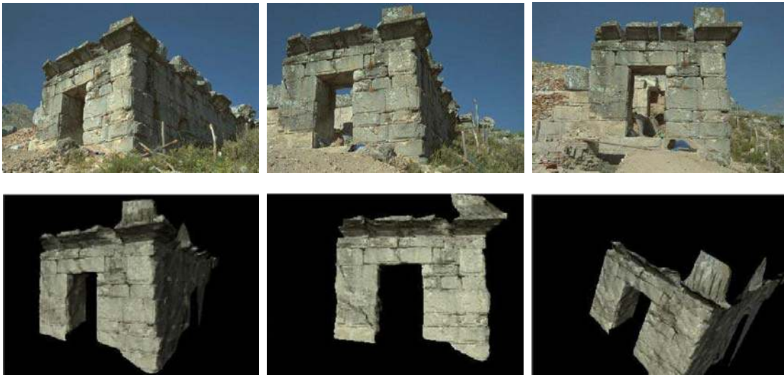
Figure 3: Top: three views of the Roman bathhouse at Sagalassos. Bottom: three views of the model constructed from 6 images of which 3 are the ones in the top row.
