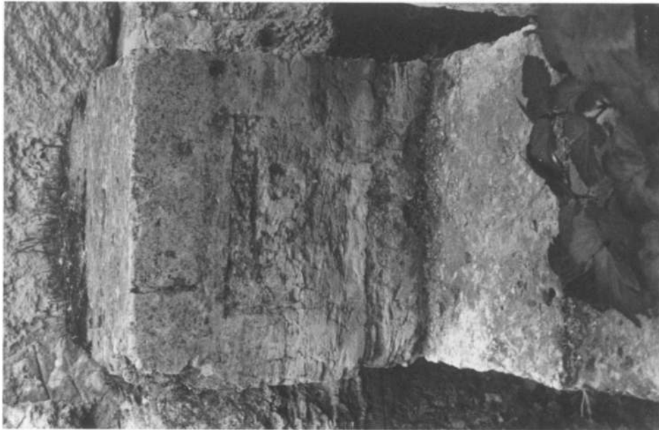
a. Anathyrosis on block of north wall 2 of the Archaic cistern. From west
