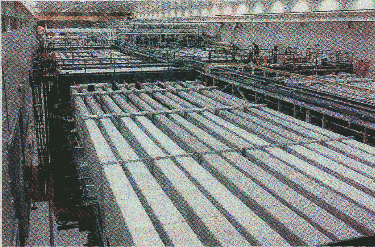
Figure 9: View of Laser Bay 2 that contains two “clusters” of 48 beams. The laser beams travel inside the beam-tubes that are prominent in the lower, center portion of the photo. Note that there are twelve flat-topped “tubes” visible across the photo; they comprise one of the clusters. Each tube consists of four independent laser beams stacked one-on-top-of-the-other giving a 4×12 array of 48 beams (this is more clearly see where the square tubes mate with the round ones near the center of the photo). The two laser bays combined contain four clusters giving 192 beams total. Work is underway to complete Laser Bay 1 by mid 2003 while commissioning shots take place concurrently in Laser Bay 2. (The workers standing on the scaffolding in the upper right corner give a sense of the scale.)
