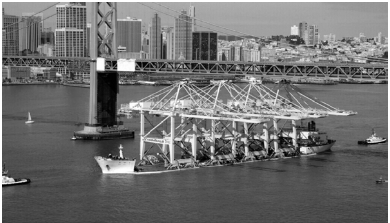
Oakland Bay Bridge, May 1, 2002
