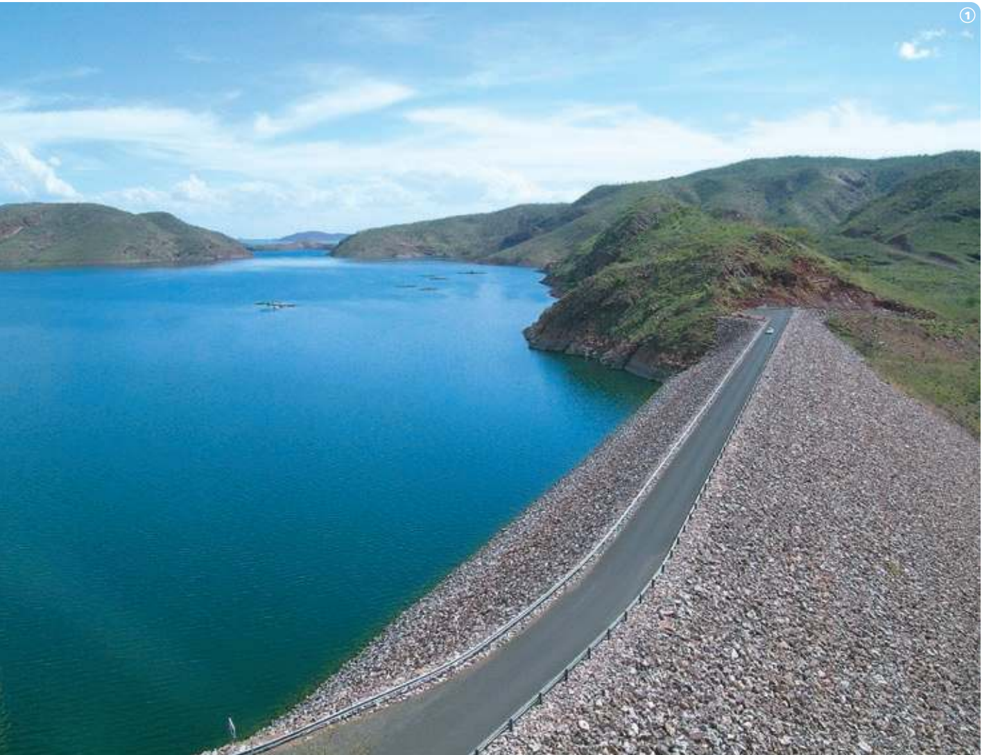
1 Ord River Dam. Photo by Stuart Blanch
