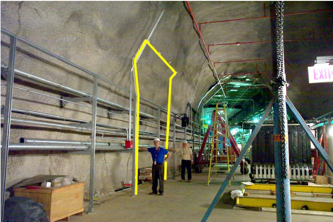
Fig. 16.3. View looking downstream in the MINOS tunnel at the location proposed for the Near Detector cavern. The infrastructure along the wall will have to be rerouted.
