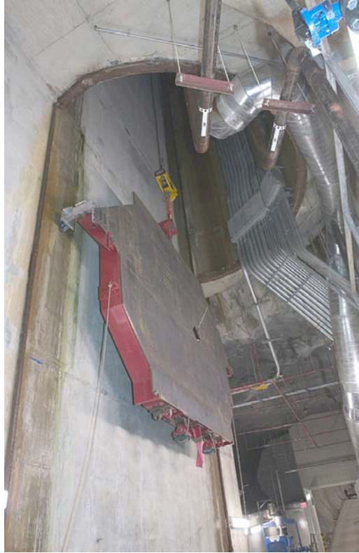
Fig. 16.4: View from the bottom of the vertical D-shaped MINOS shaft as a MINOS near detector plane comes down the shaft. The MINOS module shown is \sim 4.5 m wide by \sim 3.5 m high by \sim 0.2 m thick (including the red strong-back frame).
