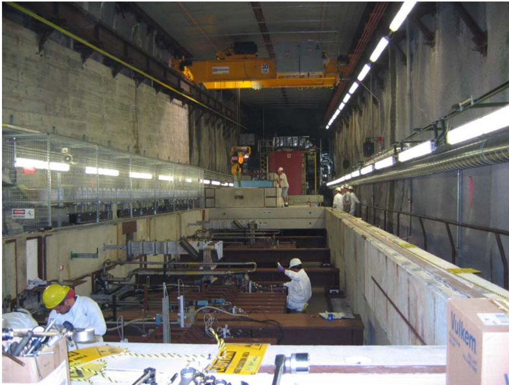
Fig 8.40: NuMI Target Hall looking downstream during a recent target repair job.
