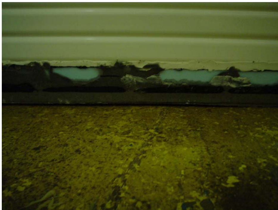
Fig. 17.115: View of grout with IPND prototype in the vertical position. The blue material is foam used to fill the gaps under the bottom horizontal extrusions of the horizontal planes.
