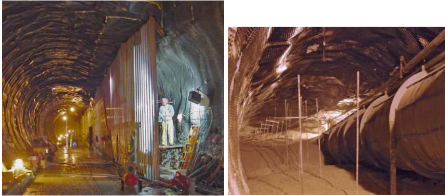
Figure 17: The NuMI Decay Pipe Tunnel. The left photograph shows the decay tunnel before the decay pipe was installed. The wall was the form for the concrete shielding and the worker shown was standing in the egress passage. The right photograph shows the installed decay pipe with concrete shielding being poured. The stiffening ribs around the pipe are also visible as well as the copper cooling lines running along the length of the pipe.
