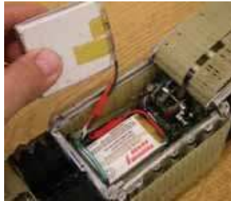
Fig. 20. The 730 mAh Li-Pol battery is in its place in Segment #5. The remaining space will be completely filled by the 2,000 mAh Li-Pol battery in the engineer's hand.
